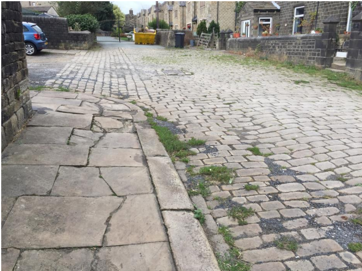
Photograph 15 Stone setts on Queen Street
