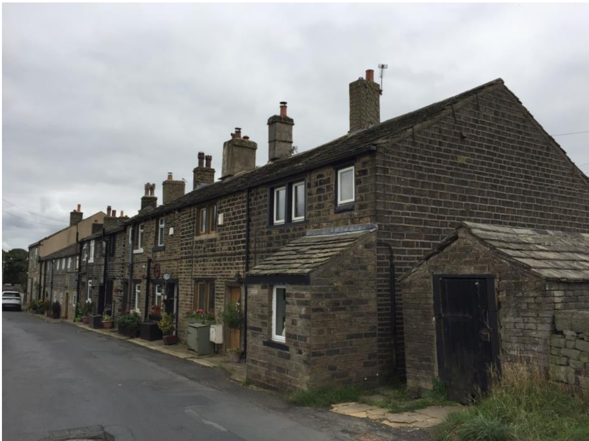
Photograph 77 Terracing at Well Head Lane/Hubberton Green Road junction
