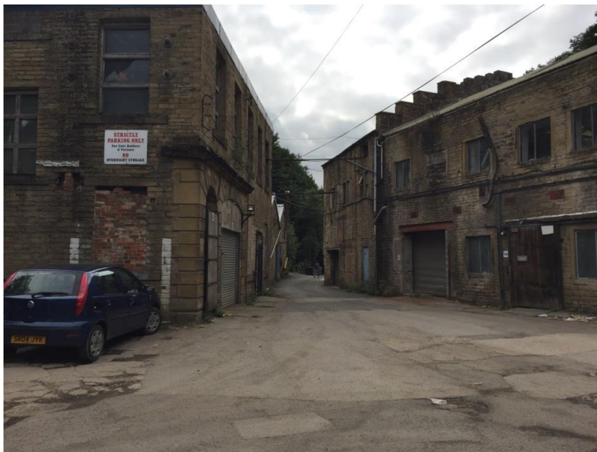
Photograph 43 Light industry and Dodge Royd woodland surrounding
