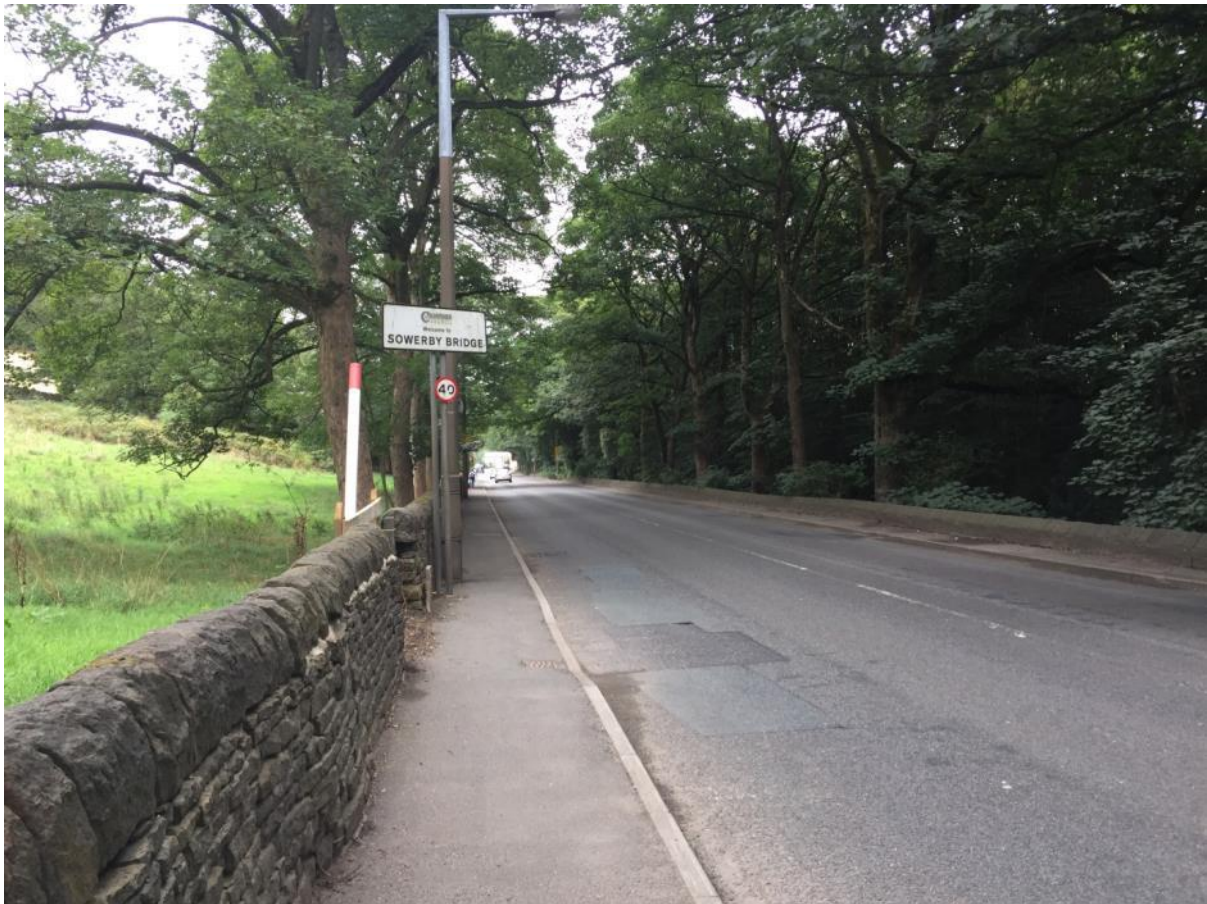
Photograph 46 The A58/Rochdale Road
