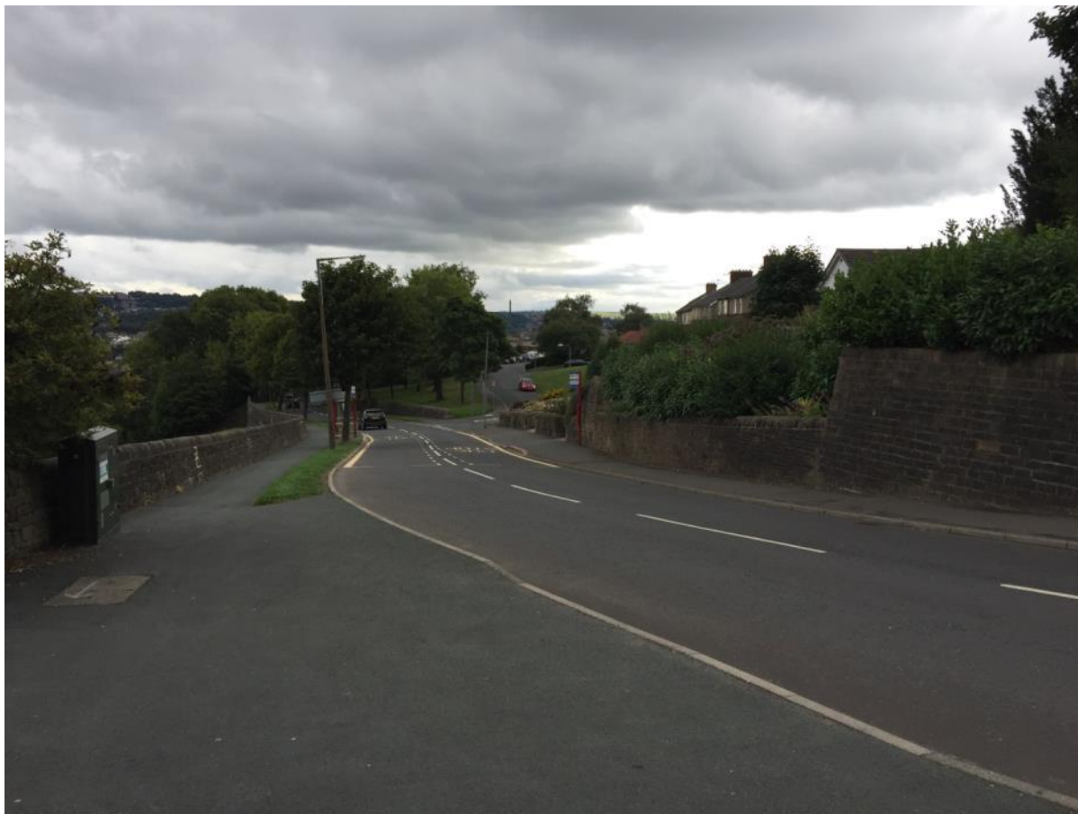
Photograph 22 Sowerby New Road
