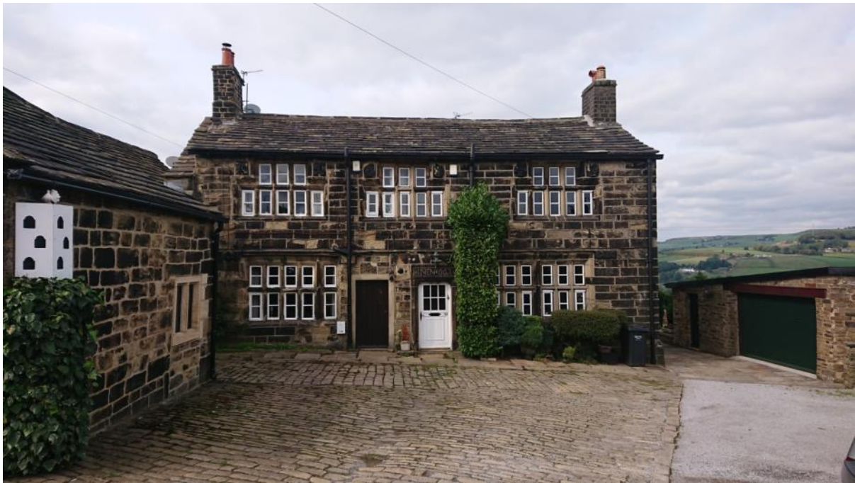
Photograph 9 No.52 and 54 Town Gate
