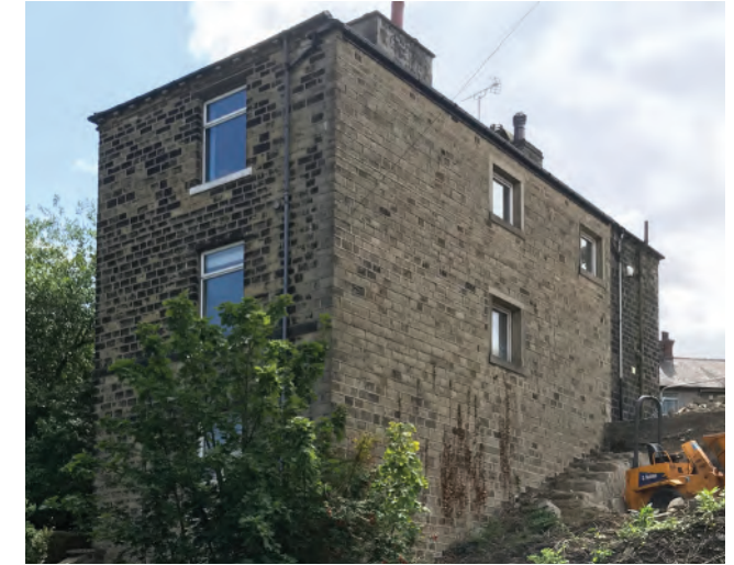
An example of a building responding to the gradient in Sowerby with a higher number of stories on one side facing towards the valley.
